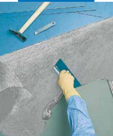
Application de Ultrabond Eco V4 SP Conductive
